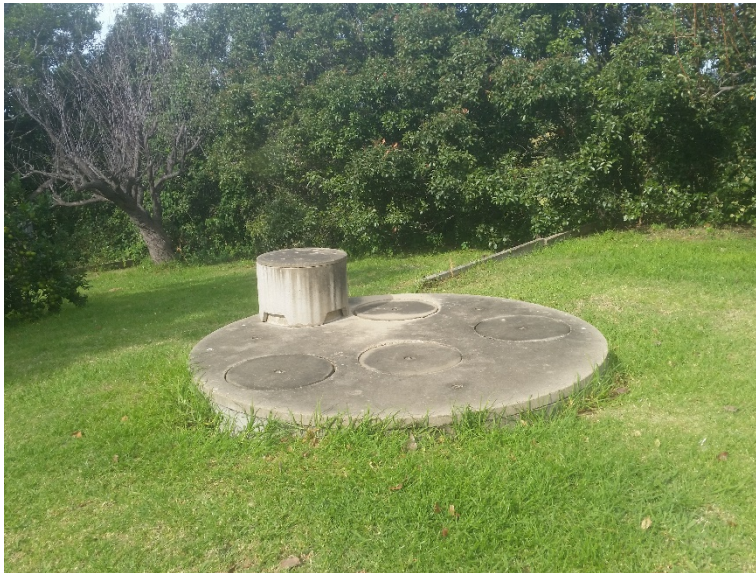
Photograph 5: Septic tank Located at Lot 1 south-east of the residential dwelling.
