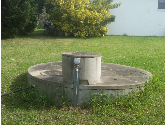
Photograph 7: Septic tank. Located at Lot 1 south-east of the residential dwelling
